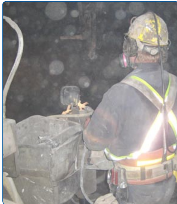
Figure 4: Spraying Shotcrete
