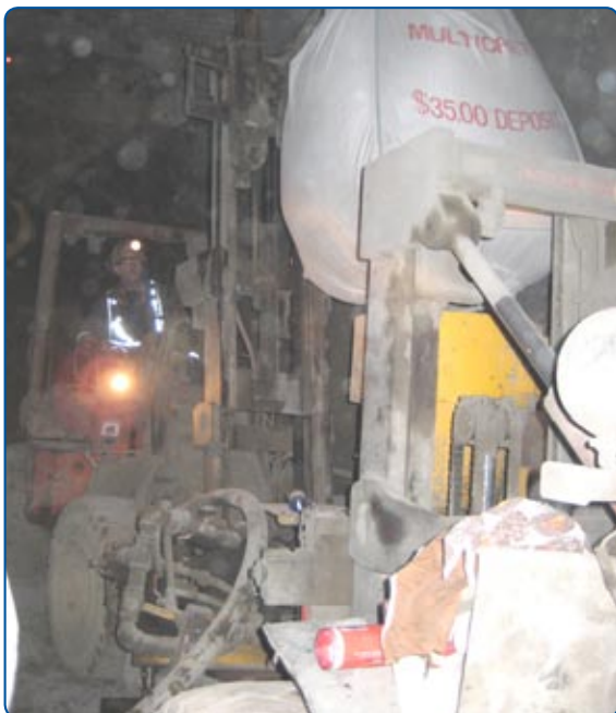
Figure 3: Preparing the Shotcrete Machine
