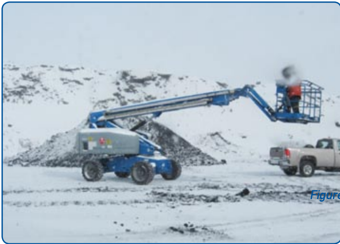
Figure 3: Elevated Work Platform
