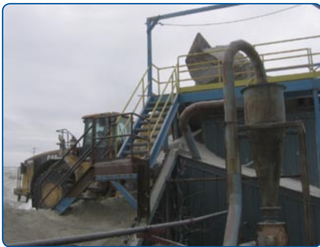
Figure 3: Loader emptying raw material into crusher
