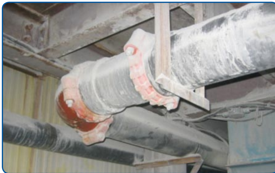
Figure 2: Workers may replace piping systems requiring ladders and/or reaching overhead
