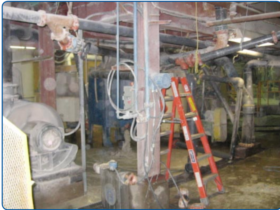
Figure 1: Ladder set up for repair of pipes
