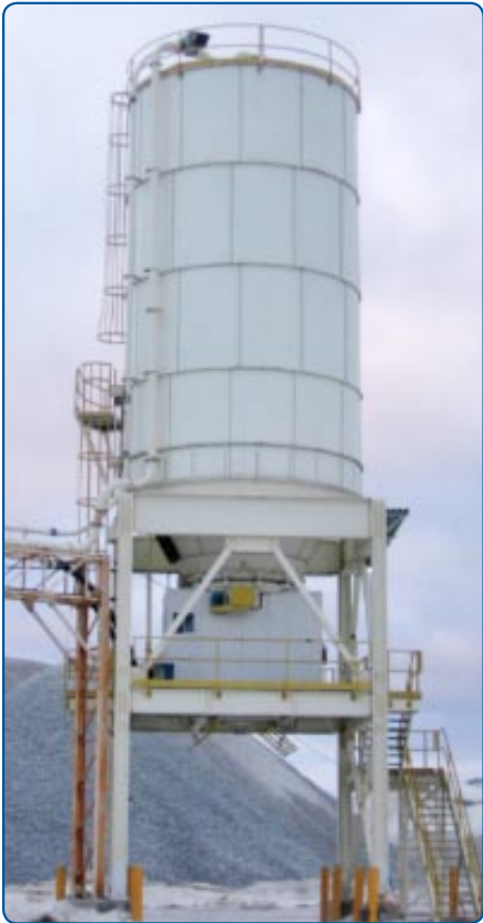
Figure 1: Storage silo for final product to be shipped
