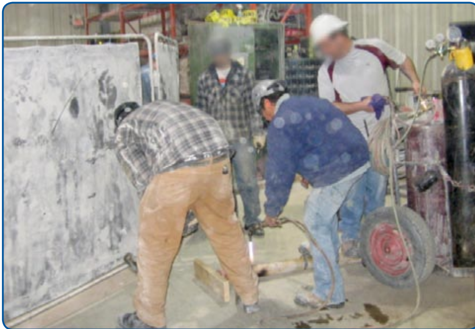
Figure 2: Worker using torch to perform repairs on a section of piping
