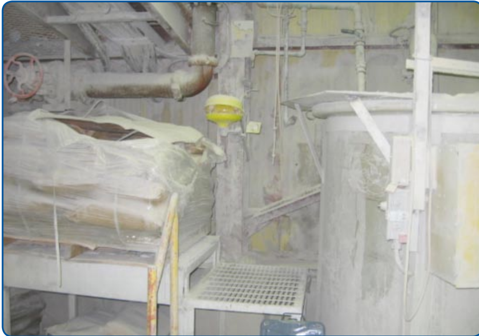
Figure 1: Dry reagent on pallet (left) to be placed in hopper (right)
